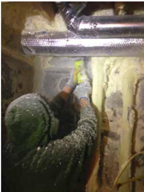
Figure 3.2 Trimming and removal of closed-cell foam using a powered brush tool.
