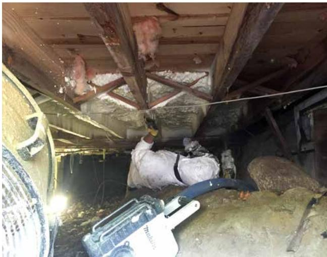
Figure 3.1 Spray foam insulation of (A) a new building (open-cell type) and B) the basement of an old house (also open-cell). The second worker in (A) is trimming the foam with a blade saw.
